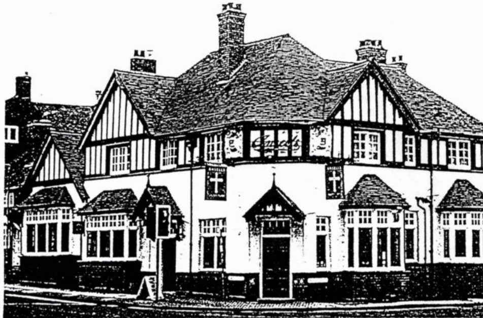
The Golden Cross in High Street, Henley-in-Arden, has finally been demolished to make way for a new development of homes and apartments. The pub, pictured above, had been closed and empty since September 1996. Allied-Domecq sold the site to Central Homes earlier this year.
