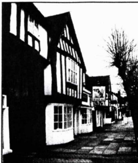
The Blue Bell before its recent refurbishment
