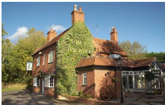
The pub. looking north from the canal bridge
